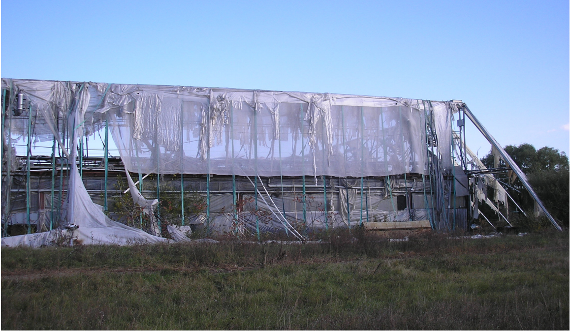
Figure 8: Current state of the Bioshelter
